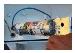
6) To assure an airtight seal, caulk around wires and cables, coating entire plug surface with sealant.
