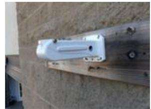
Mounting to wall requires four user supplied fasteners. Mark pilot holes for four (4) mount holes either by marking with base, or using template guide on back page of this manual. Drill pilot holes and bolt arm to wall securely. Four holes on S-Type arm will accommodate up to 5/16" diameter bolts. Always assure there is strong backing material & the proper strong & secure to anchoring into aggregate material of wall is made.
