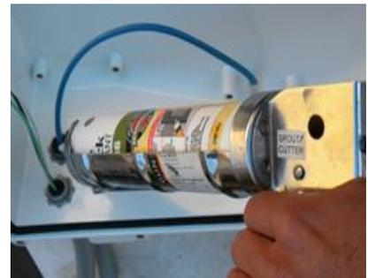
6) To assure an airtight seal, caulk around wires and cables, coating entire plug surface with sealant.
