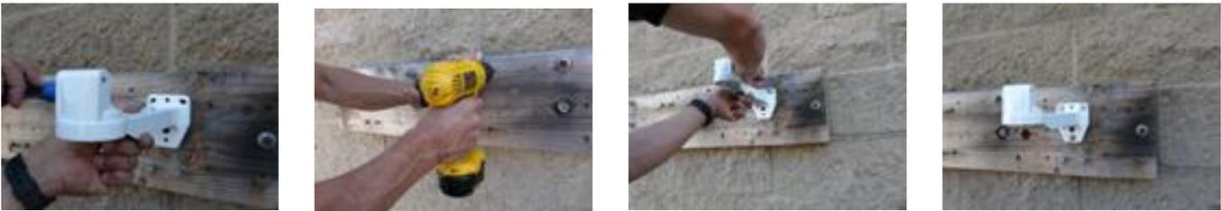
First Mark Holes in desired location, using wall mount, or template guide on last pages of this manual. Pre-drill Pilot holes for anchoring fasteners in marked positions, then fasten mount to wall securely as shown.
