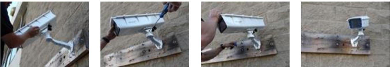
Using two side screws removed in first step, re-assemble Tilt bracket to wall mount as shown. Loosen & then re-tighten screws for Pan & Tilt adjustment to arrange housing to desired viewing angle. Securely tighten all fasteners to final position. Install Power and Data cables as desired thru ports on rear of S-Type enclosure. Always create a "drip-loop" for wire or cable that comes from above enclosure.
