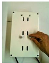
Then install the lower mounting bolts 3/8"-18 x 1" on bracket, leaving hex head protruding about 3/8"
