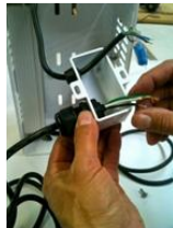
Then, Pull customer provided wiring first thru one of the four round cable ports on metal bracket, then thread cable thru cable gland port on small electrical box
