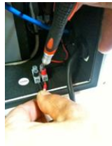
Using a small flat blade screw driver, secure wires to color coded terminals as shown
