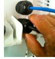
Securely tighten seal nuts on all cabling for proper seal and cable strain protection
