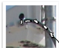
Arrows illustrate air flow within conduit when wire feed is not sealed within enclosure
