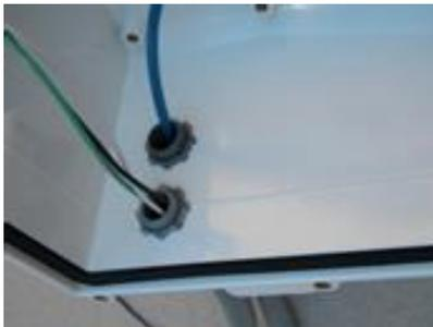
1) Pull wires to final installed length.
