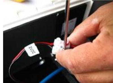
Pull power and Data cables into housing thru Cable Gland strain relief seal ports near rear of S-Type enclosure. Strip back wires on Low Voltage 12VDC power cable brought into enclosure, observing DC polarity.
