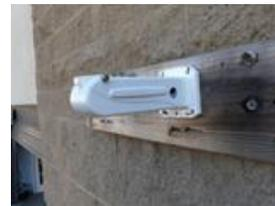
Mounting to wall requires four user supplied fasteners. Mark pilot holes for four (4) mount holes either by marking with base, or using template guide on back page of this manual. Drill pilot holes and bolt arm to wall securely. Four holes on S-Type arm will accommodate up to 5/16" diameter bolts. Always assure there is strong backing material & the proper strong & secure to anchoring into aggregate material of wall is made.
